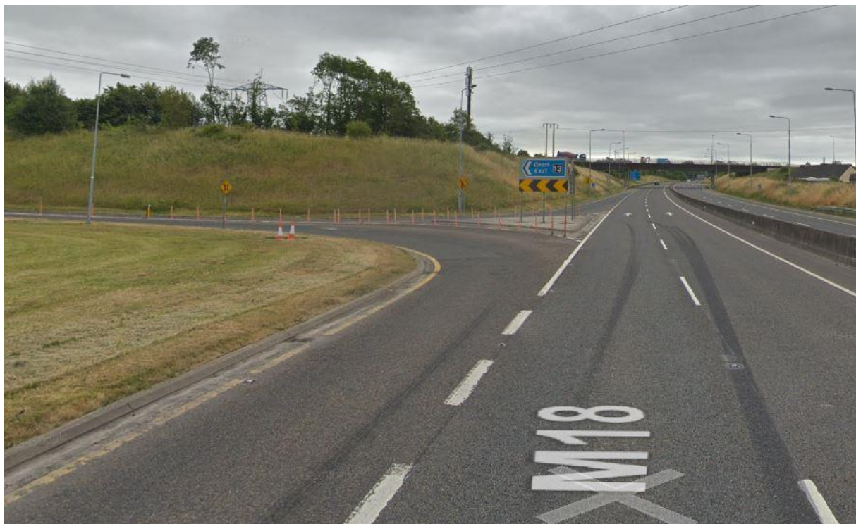
Figure 21 - Junction 13 south bound exit
