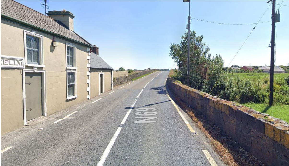
Figure 26 - Ferry Bridge on the River Maigue facing east
