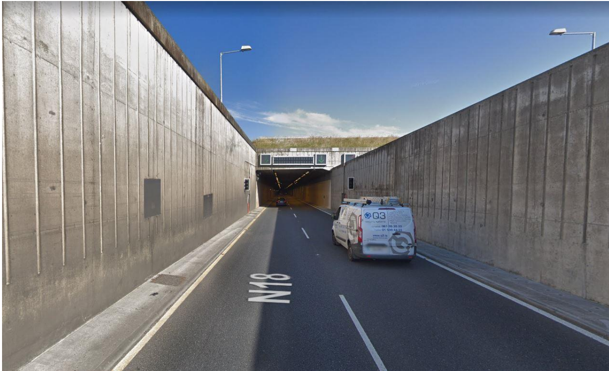
Figure 32 - N18 Limerick Tunnel entrance north bound
