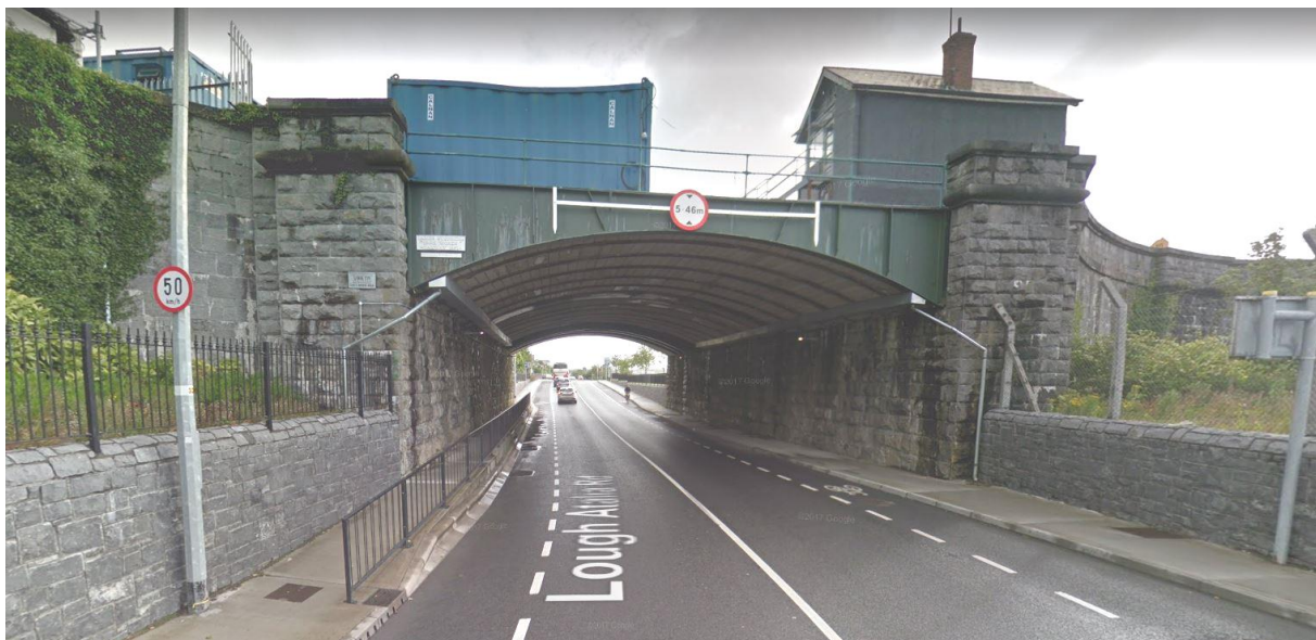
Figure 8 - Railway bridge on Lough Ataile Road
