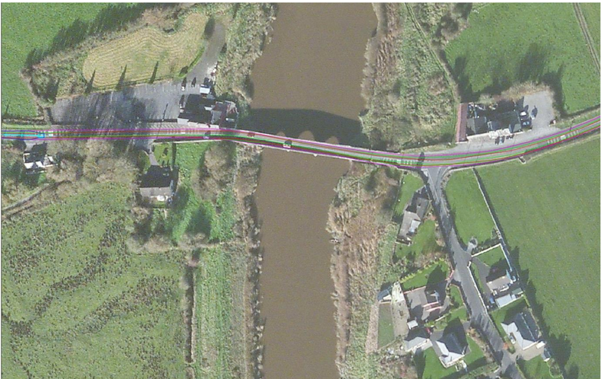
Figure 27 - Ferry Bridge on the River Maigue - swept path
