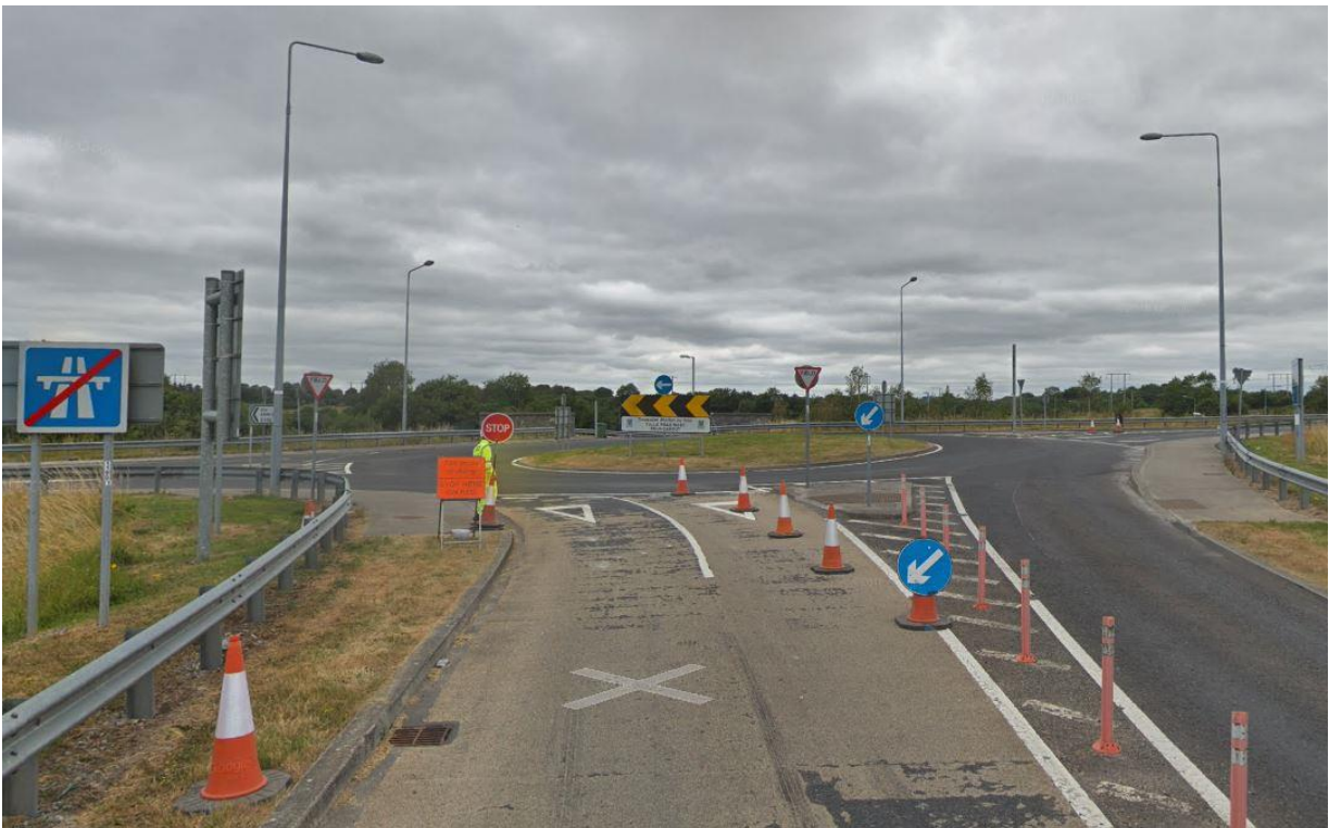
Figure 36 - Junction 13 north bound, approach to west roundabout
