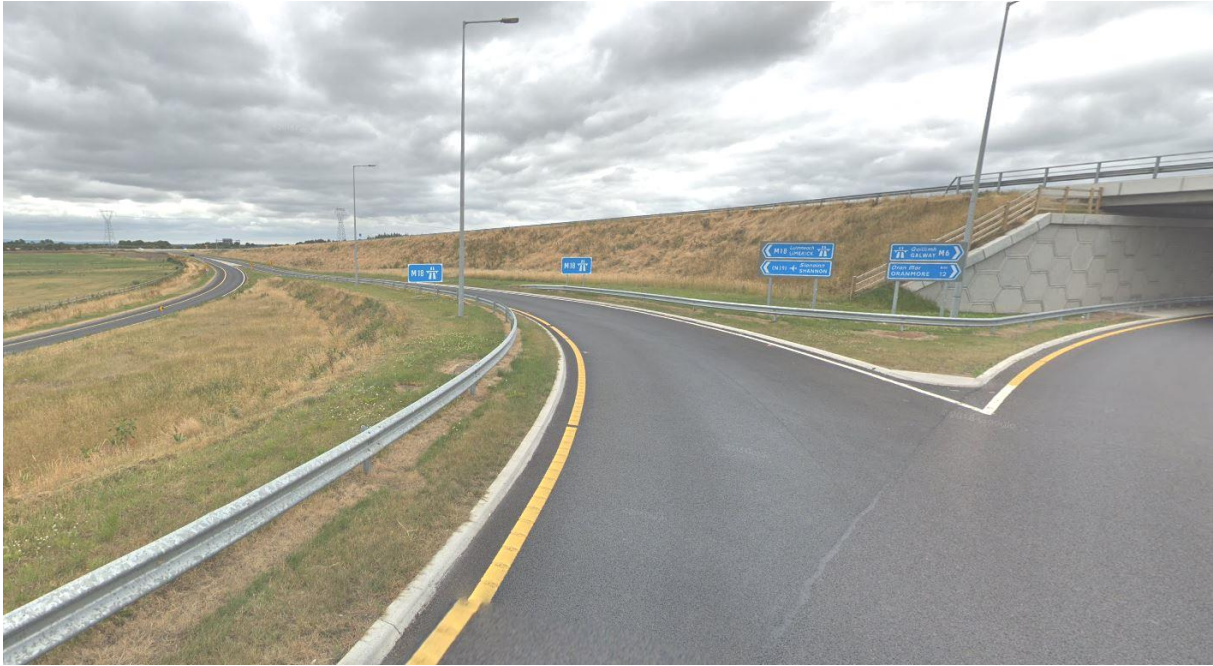
Figure 18 - Exit to M18 from M6 / M18 interchange
