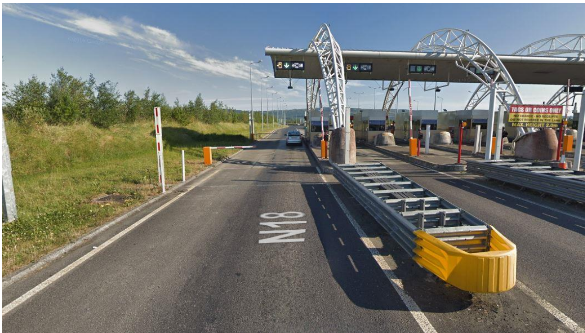
Figure 33 - N18 toll plaza north bound
