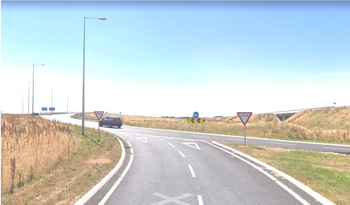
Figure 16 - Yield line at entry to M6 / M18 interchange
