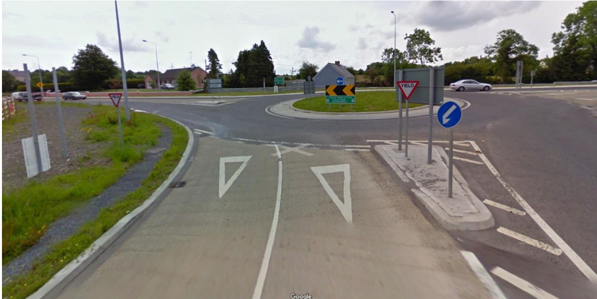
Figure 22 - Junction 13 south bound roundabout
