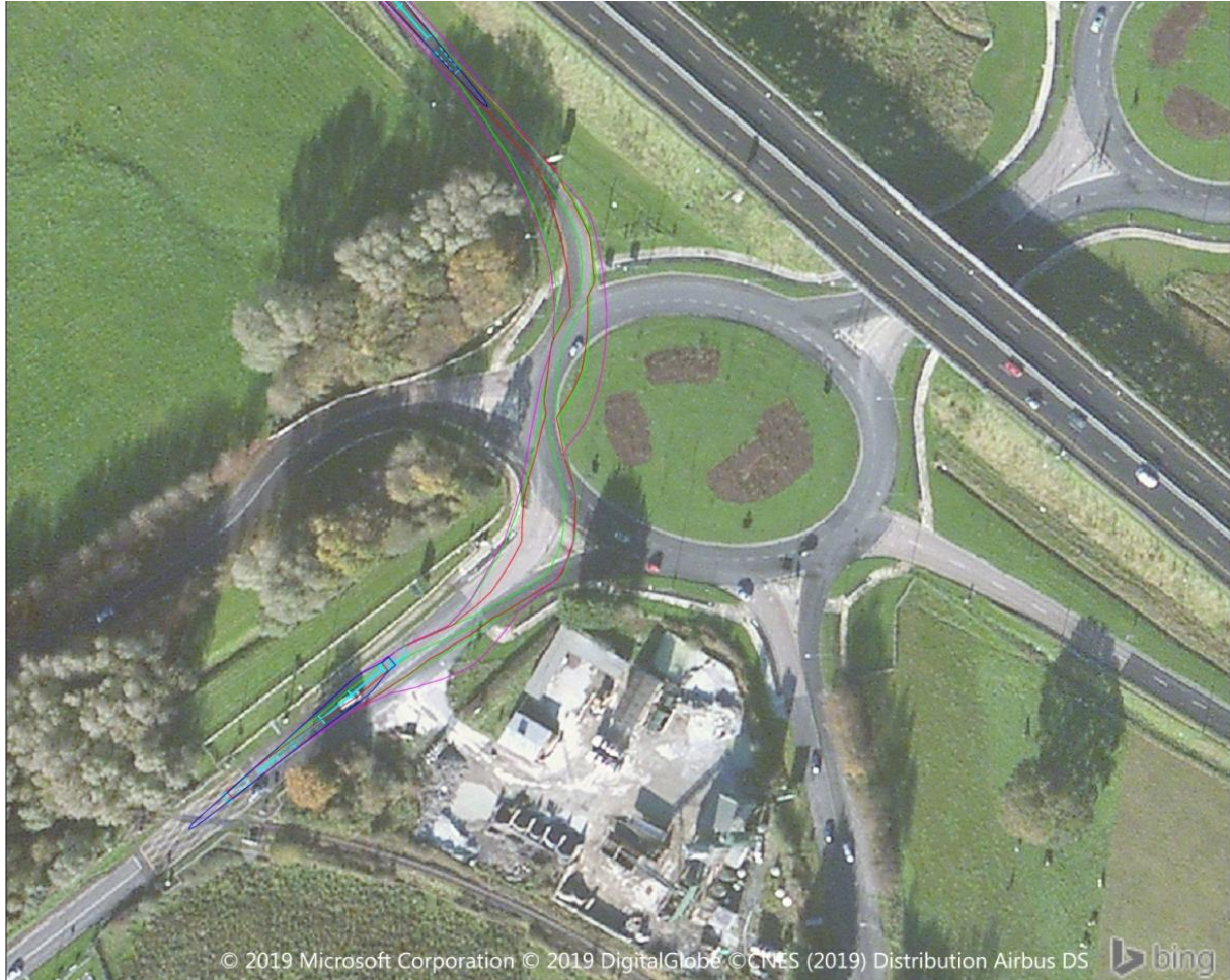
Figure 31 - N69 Dock Road roundabout to N18 on ramp
